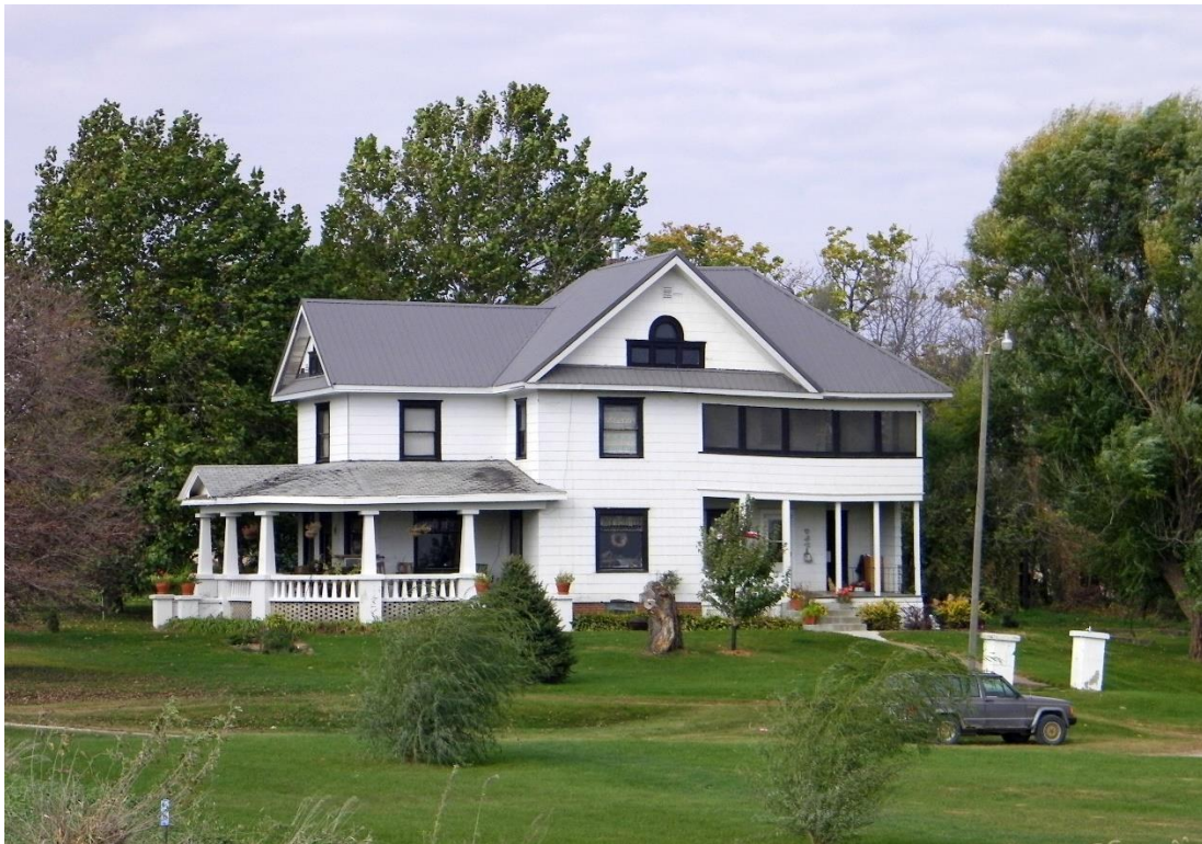
The Christian Gensicke Farm, 2010. The house has been modernized and expanded since it was first built.
